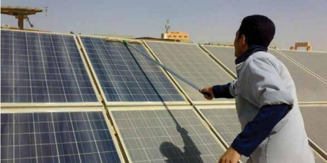
When inspecting the solar panels, the bearing structure should also be checked. Two main things to pay attention to are: threaded connections - whether there is corrosion and construction safety check - whether it is firmly mounted.
