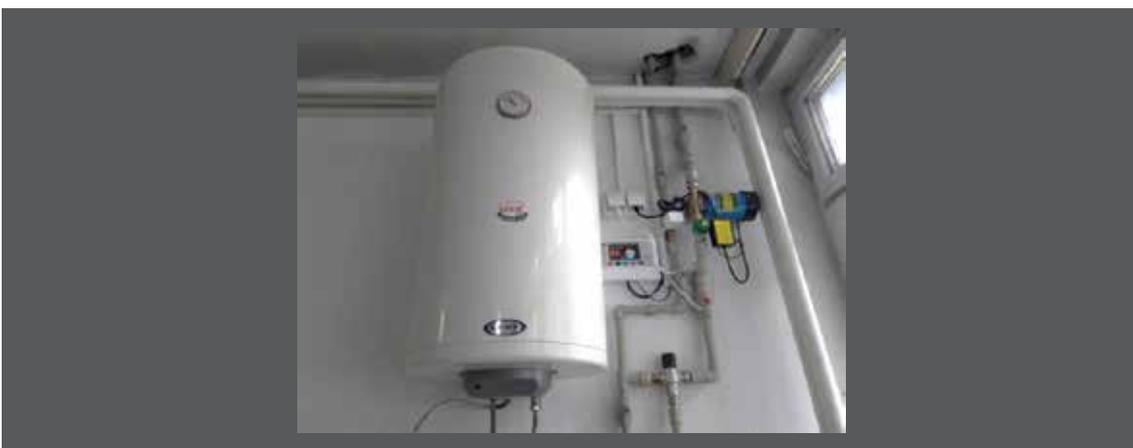
Maintenance of these systems is the same as in the previously described thermosiphon systems. There is only one difference - if the system does not have a leakage pressure of the sanitary hot water it is necessary to check the condition of the sensor (indicator) and the valve that regulates the filling of water in the boiler and the operation of the pressure boosting pump.
